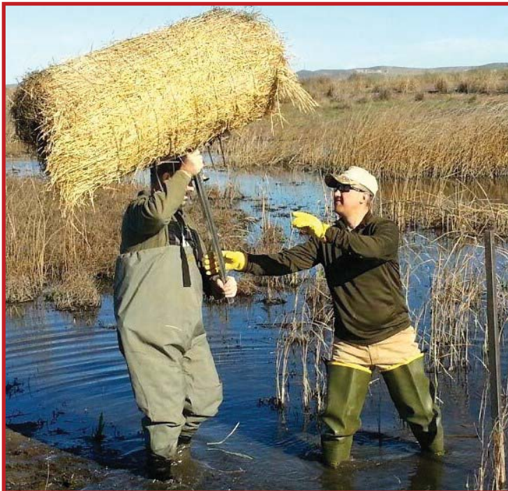
Scott Honeycutt hands Abel Cortina the top portion of the Nest Tube to slide into the already embedded angle iron steel sleeve to Abel's left.
